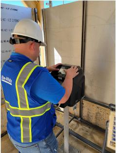
Figure 1. FLEXFLO® Peristaltic Pump Being Programmed at a WWTP.
