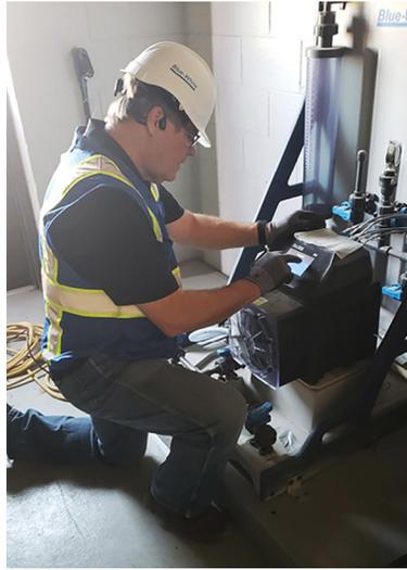
Setting the Pump up using the touchscreen display
